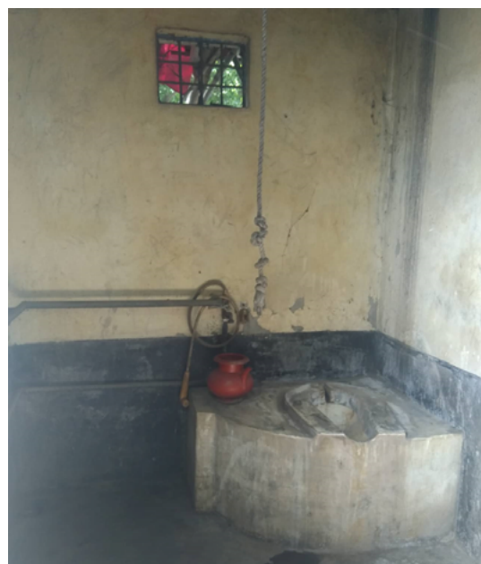
Figure: Disabled friendly toilet structure in Kallyanpur slum
